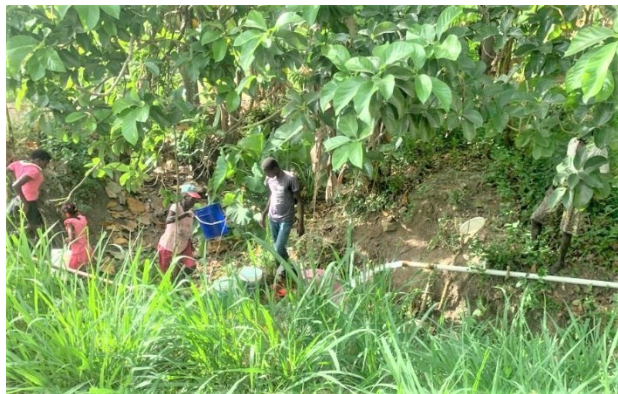
Repairing Water Line
