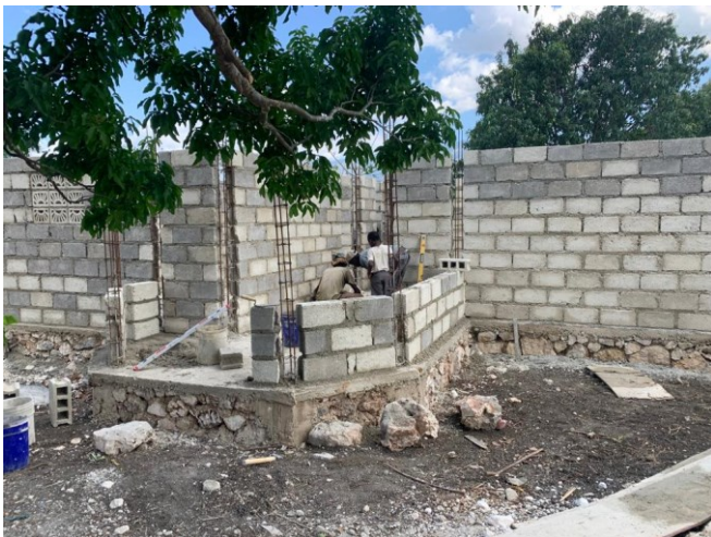
Day 28 Building the Walls
