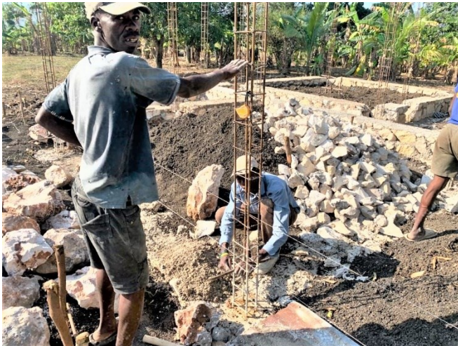
Day 17 Working on the Foundation
