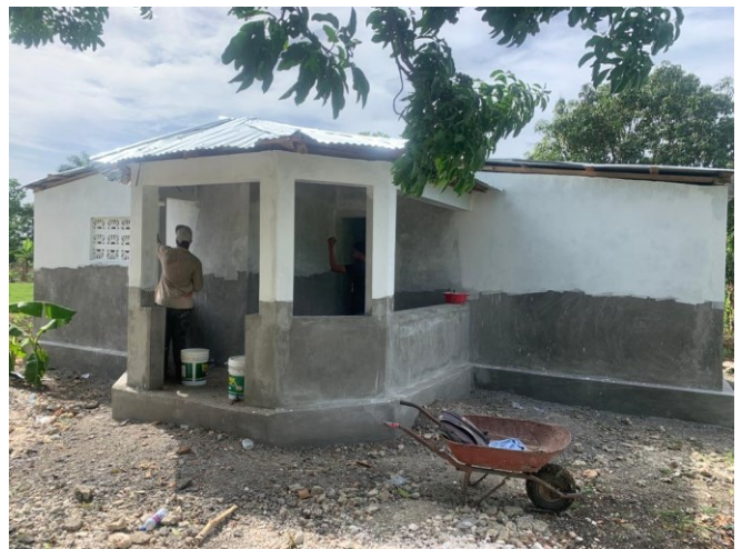
Construction Day 75 Painting
