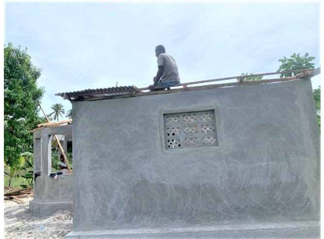
Construction Day 72 Putting on the Roof
