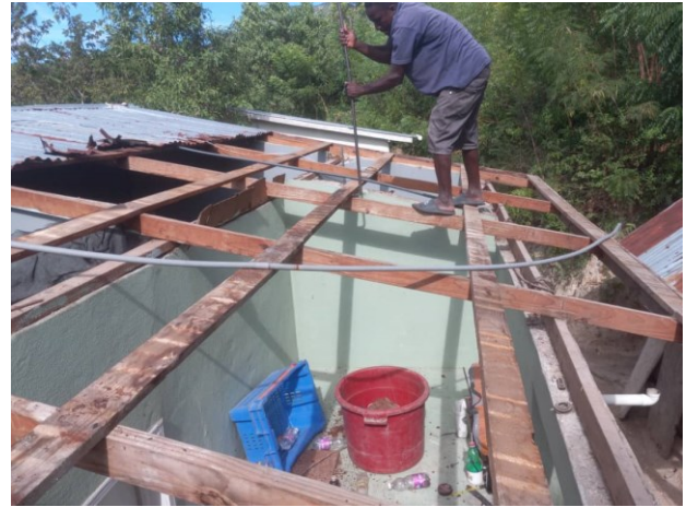
Repairing Roof of Christella Julsaint
