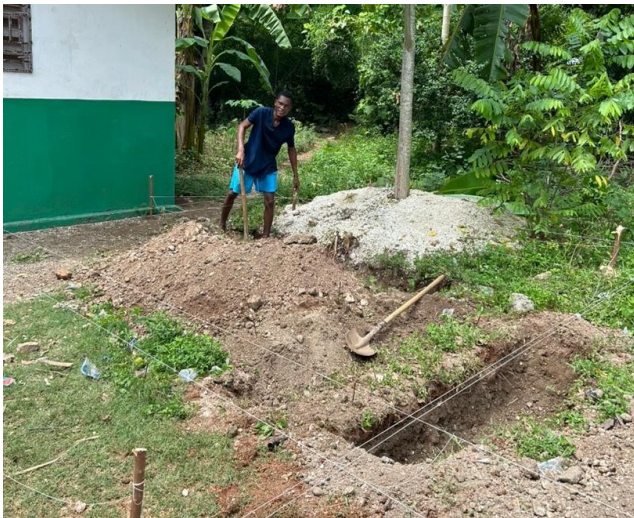
Clinic Toilet Begins
