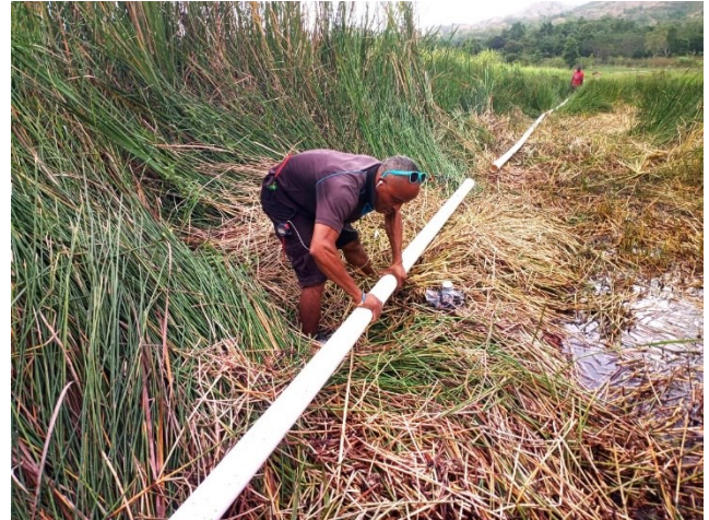
Assembling the Pipe
