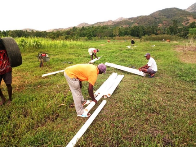
Laying out the Pipe
