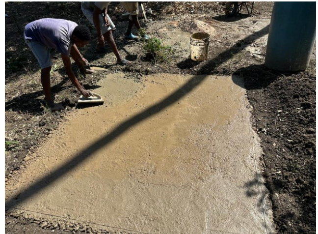
Platform for Well Drilling
