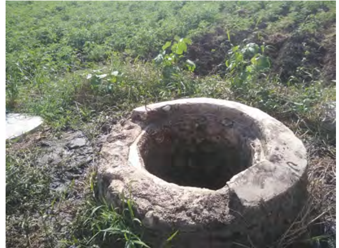
Nearby Country Well Without a Pump
