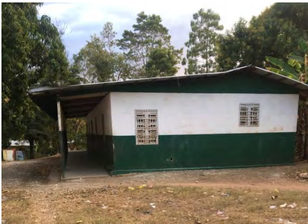
The Clinic Building
