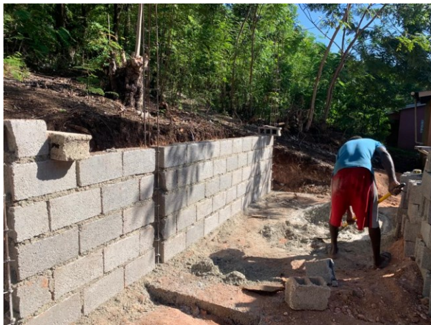
Building the Structure
