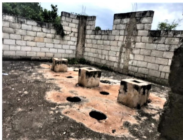
Present Public Latrine
