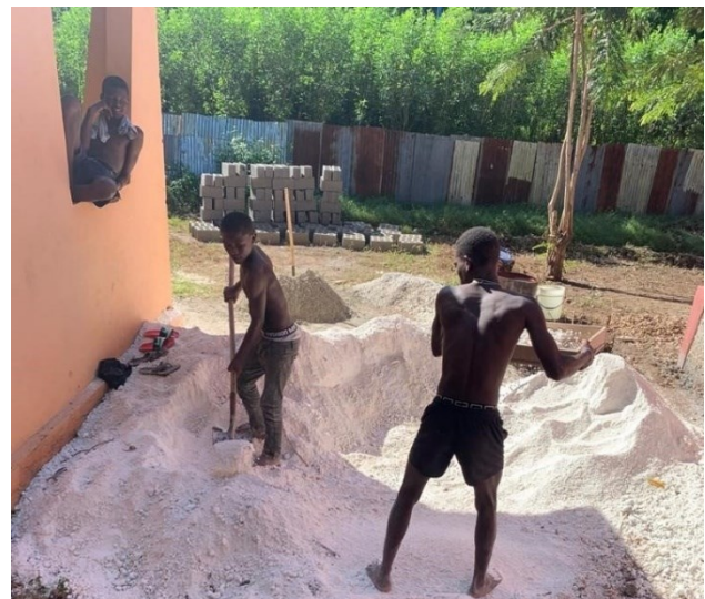
Starting to Build Near Grain Mill
