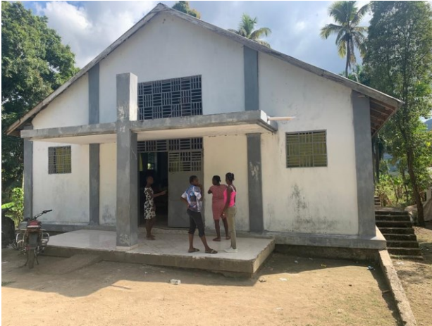
The Methodist Church of Fond Doux
