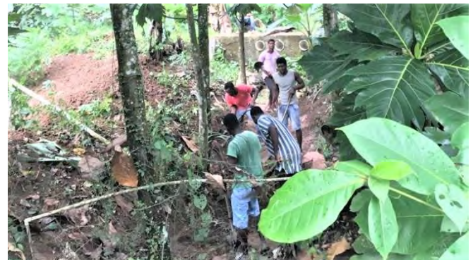
Fixing Drainage Problem
