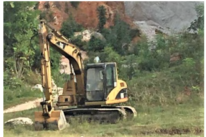
Power Shovel to Remove Hill
