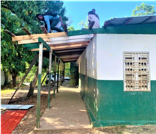
Repairing the Roof of the Clinic Building
