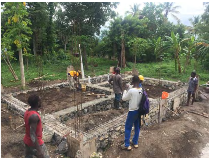
Day Three Construction
