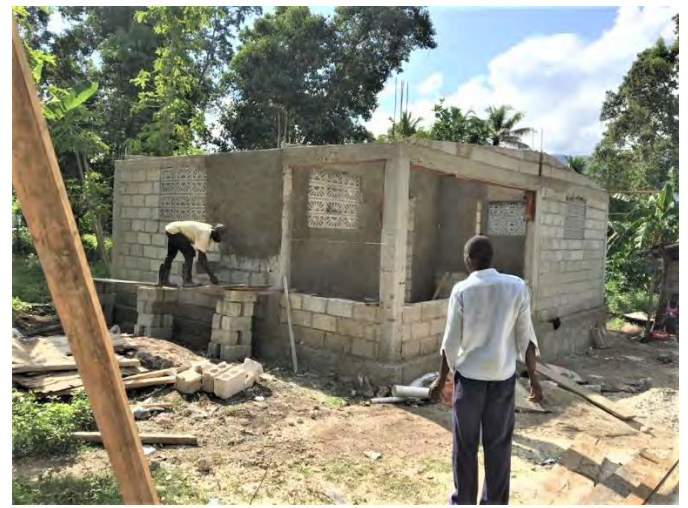
Day Nineteen Stucco Construction
