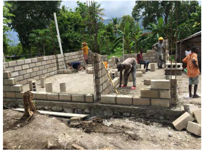
Day Six Construction
