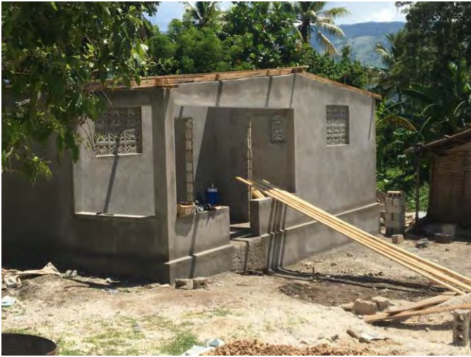
Day Twenty-six Roof Construction
