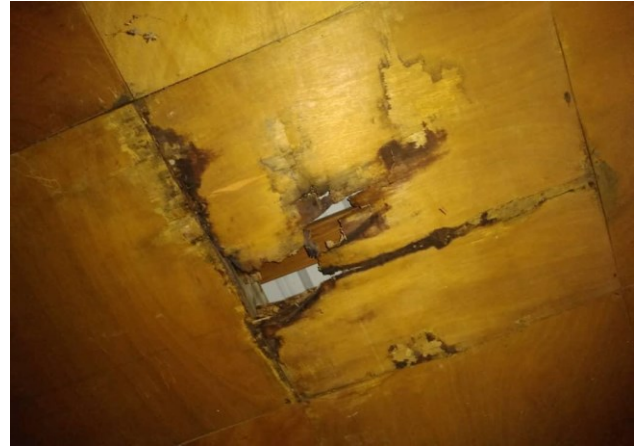
Ceiling in the Pharmacy
