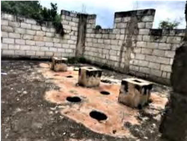
The Existing Latrine
